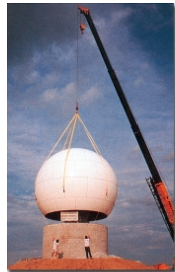
Strong, lightweight FRP/Composite domes use self-supporting sandwich construction to protect sensitive electronic equipment from the Sahara to Antarctica while remaining transparent to the electromagnetic signals.
