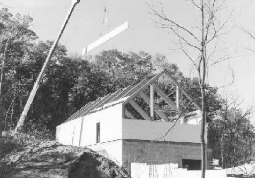
Fig. 48 All-composites skeleton. (Courtesy of Strongwell Company)
