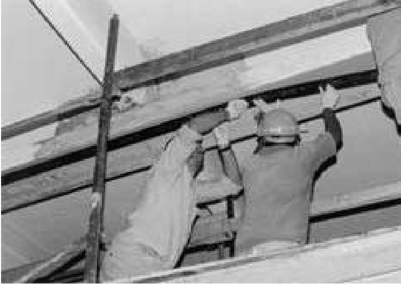
Fig. 5 Reinforced concrete beam strengthening applications using precured composite strips. [Courtesy of Structural Composites Construction Inc. (SCCI)]
