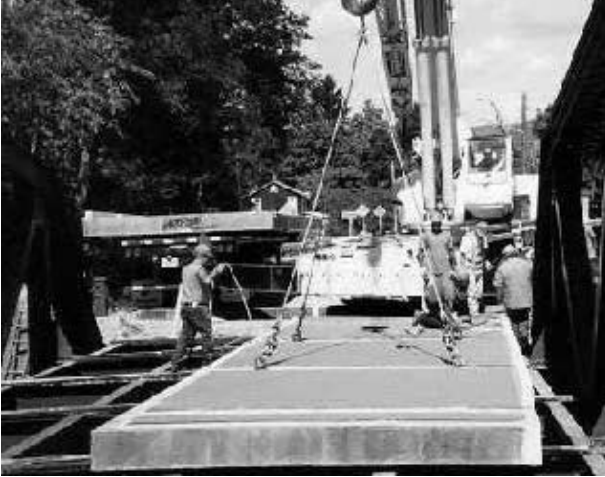
Fig. 51 Installation of all-composite bridge deck of NY 367 over Bentley Creek, Chemung County, New York (2000). (Courtesy of New York DOT, Region 6, Hornell, NY)
