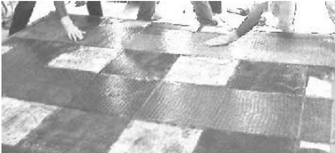
Fig. 11 Structural strengthening of unreinforced concrete slab-on-grade using polymer composites. [Courtesy of Structural Composites Construction Inc. (SCCI)]
