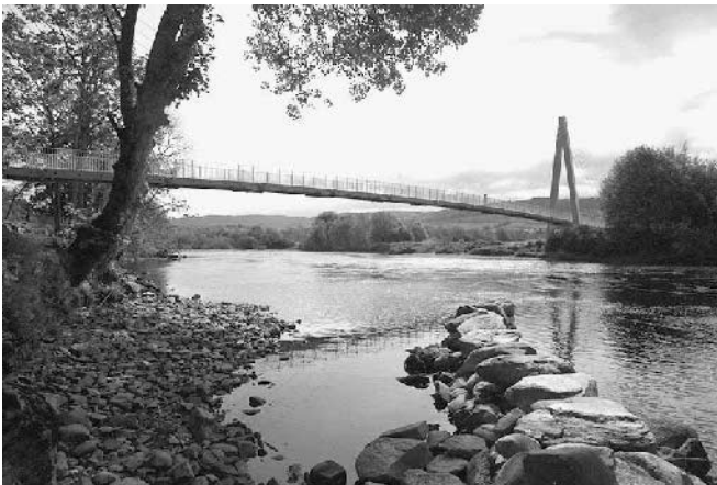
Fig. 56 Aberteldy all-composites cable-stay bridge. (Courtesy of Strongwell Company)
