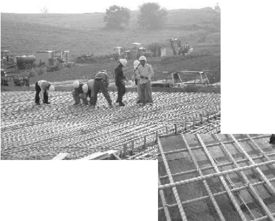
Fig. 33 FRP composite reinforced bridge deck. (Courtesy of Hughes Brothers Company)
