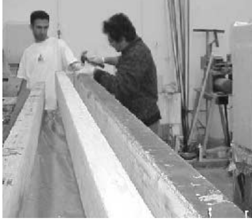
Fig. 15 Structural strengthening of glue-lam wooden beams using carbon/epoxy sandwich composites. (Courtesy of Sigma Composites, LLC)
