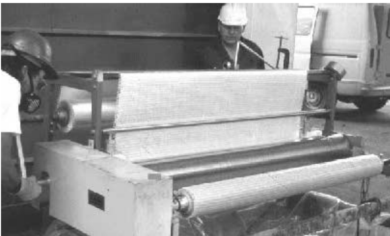
Fig. 20 Use of automated saturators is the preferred method for wet lay-up repair process. (Courtesy of Fyfe Co. LLC)
