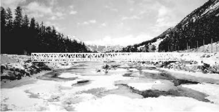
Fig. 58 Pontresina all-composite truss bridge constructed in Switzerland in 1997. (Courtesy of Fiberline Composites A/S)
