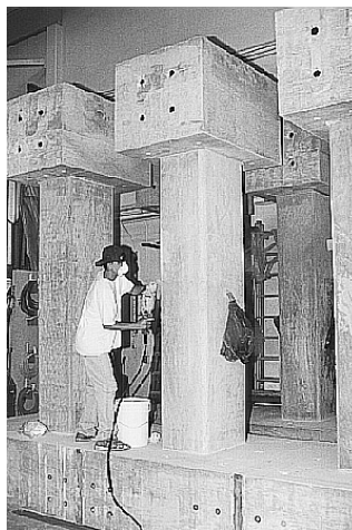
Fig. 27 Minimum radius of 0.75 in. (20 mm) for noncircular columns is required before the application of FRP composites. (Courtesy of Professor M. Haroun, University of California, Irvine)
