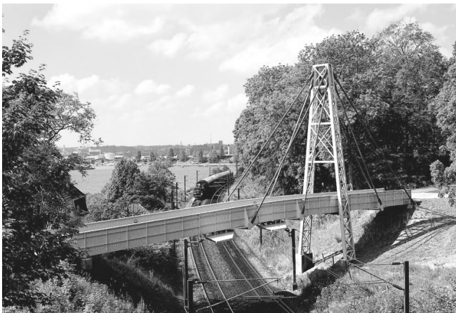
Fig. 57 Fiberline all-composite cable-stayed in Denmark. (Courtesy of Fiberline Composites A/S)
