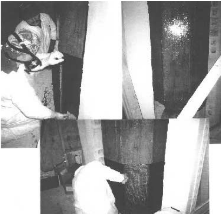
Fig. 1 Seismic upgrade of columns using composites. [Courtesy of Structural Composites Construction Inc. (SCCI)]
