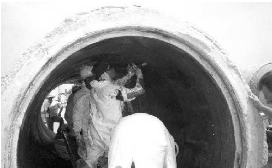
Fig. 12 Strengthening of reinforced concrete pipes using polymer composites. [Courtesy of Structural Composites Construction Inc. (SCCI)]
